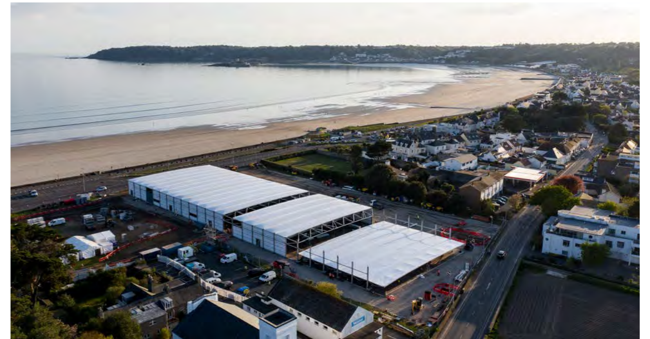
We constructed the Jersey Nightingale Hospital in just four weeks
