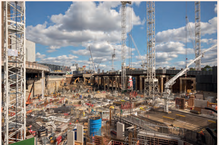
Battersea Power Station Phase 3a
